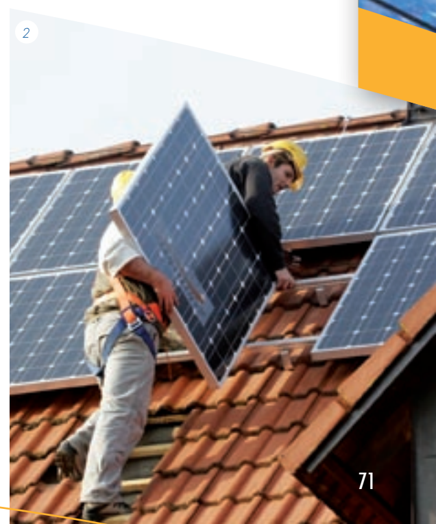
2. Installers setting up a roof-top residential PV system in Germany © SHARP ELECTRONICS (EUROPE) GMBH 2010
